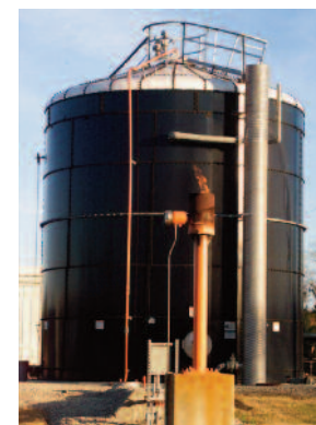
Figure 9. Fixed-film digester. (Courtesy of Ann Wilkie, University of Florida—IFAS).
