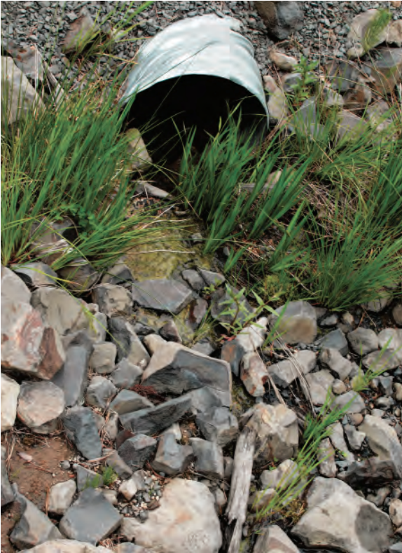
Stable areas have rocks, slash, or vegetation at drainage outlets.
