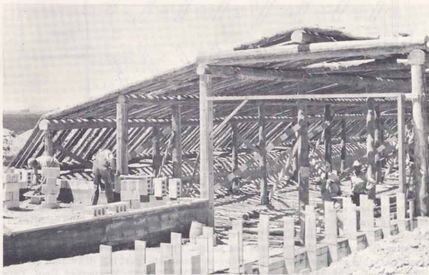
Figure 2. Typical construction of supported roof, pole-type, partially below ground potato storage.
