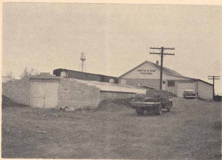
Figure 4.—A small two-story packing plant built in conjunction with a potato storage cellar.
