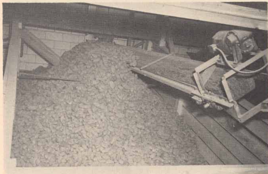
Figure 12.—The Figure 10 bin being filled with potatoes. The rear of the bin fills first and then the tubers are distributed forward by the inclined belt. A belt conveyor under the bin moves the potatoes out of storage. The only labor required to operate the system is that of starting and stopping the drive motors.
