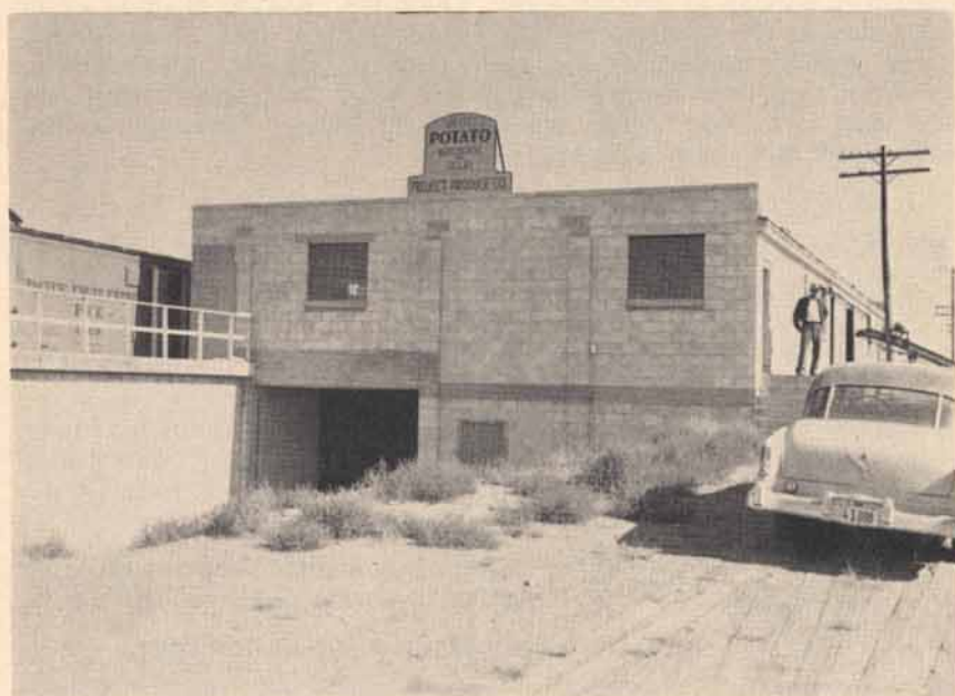
Figure 2.—Double-story, concrete block potato packing plant of the type used most widely in Idaho.
