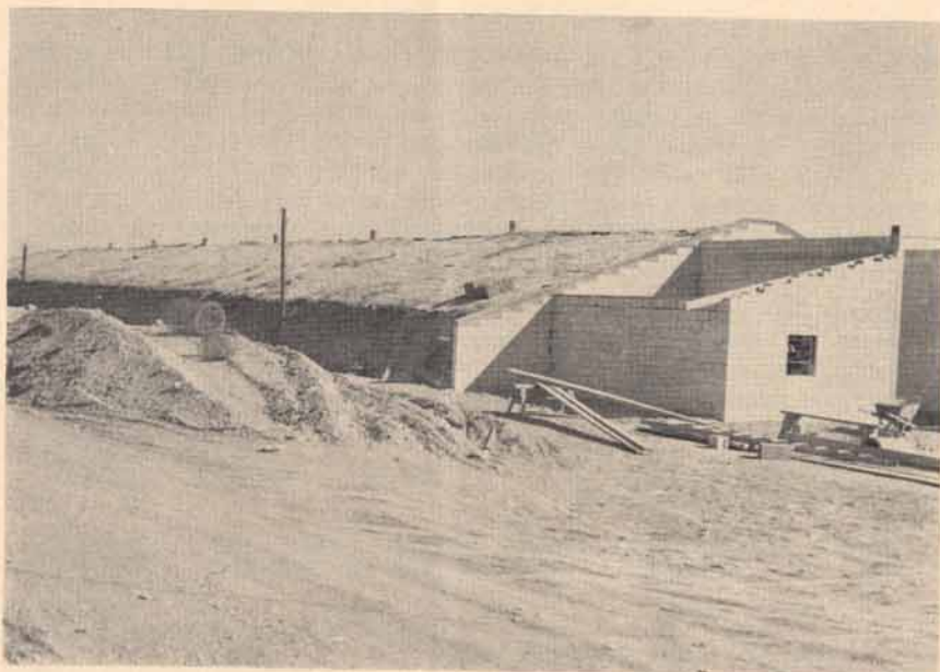
Figure 3.—Cellar-type packing shed with concrete block ends and straw roof and sides. Roof will be covered with a light layer of soil.
