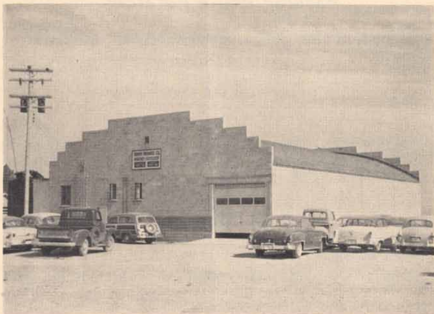
Figure 1.—Single-story, trussed roof packing plant of recent design.
