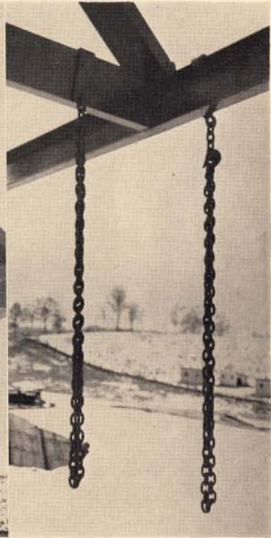
Figure 3.—Load anchor chains are attached to brackets on the channel iron frame. The free end of the anchor chain is equipped with a grab hook for quick and easy fastening to the load.
