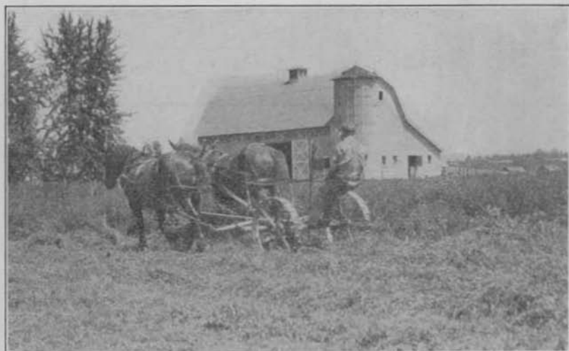
Cutting Alfalfa at the Sandpoint Substation
