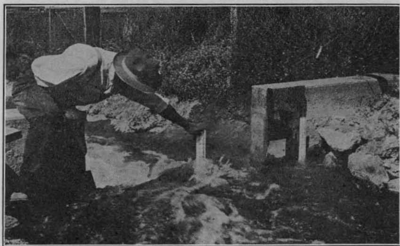
Figure 16—The velocity of approach too high.
