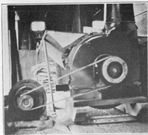
Blower type elevator located at farm storage plant and operated by three horsepower electric motor.
