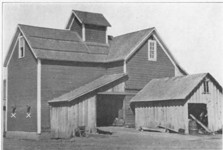
Note the grain chutes (marked X) used for loading the truck boxes when the wheat is to be hauled to market.
