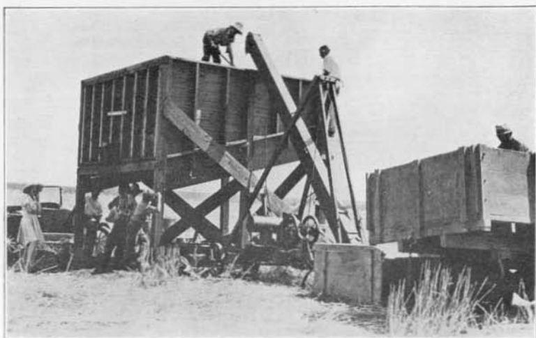
Intermediate field bin using sloping floor and side grain chute.
