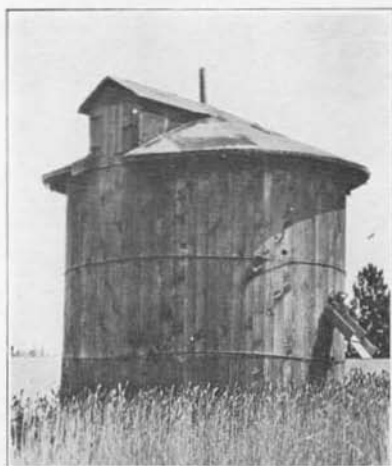
Field storage bin. Note gravity chute on the side.
