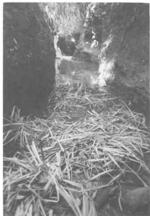
Brush and debris in the stream.
