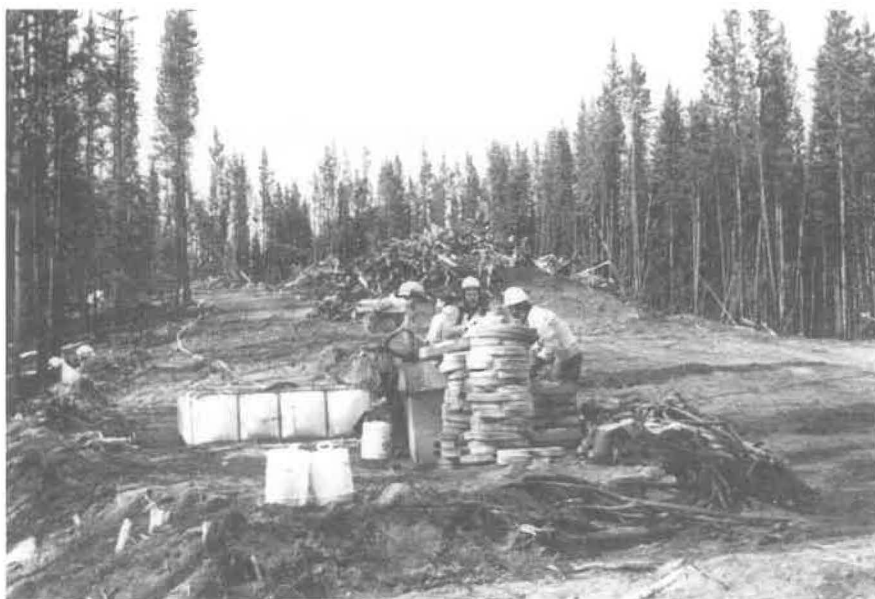
Staging areas are widened for buses, equipment, storage, and as safety areas for firefighters to retreat to. These areas require rehabilitation immediately after the fire is put out.
