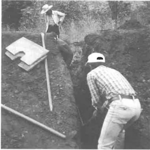
Pancho and a farmer install drainage pipe in an earthen dike
